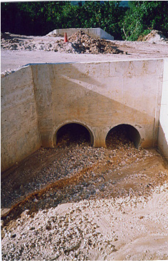
Dual culverts can often help mitigate heavy rainfall.
