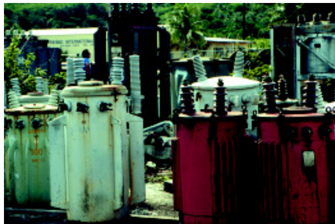
Dumps containing old electrical transformers (which are filled with highly toxic chemicals) are still being found in the CNMI.
