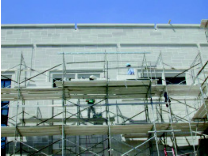
Economists group together industries such as building construction and building services.
