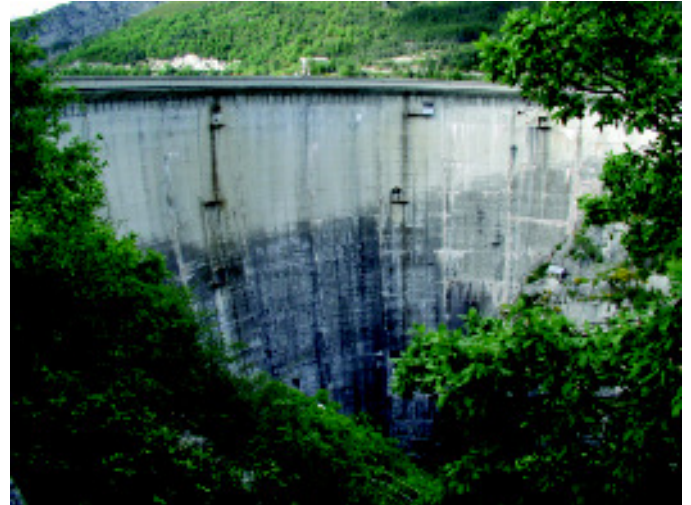
Dams can block migration routes up rivers and thus eliminate much of the habitat that fish need to reproduce.
