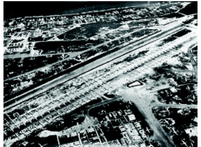
To prepare Saipan for the arrival of the B-29 Superfortress, US forces built two large runways, 186 buildings, and a special road between the airfields and a nearby coral quarry.
