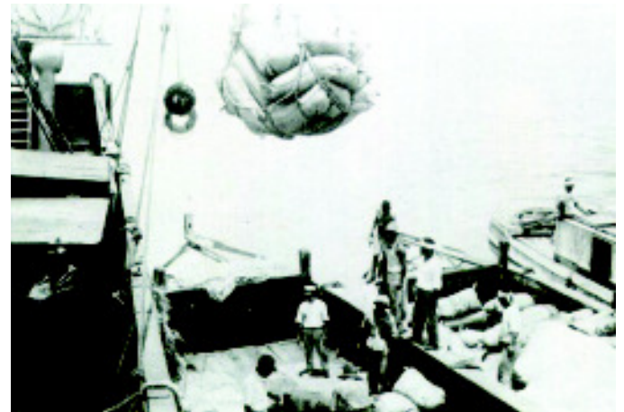
The new harbor allowed ships with a draft up to 28 feet to pull alongside the new jetties.
