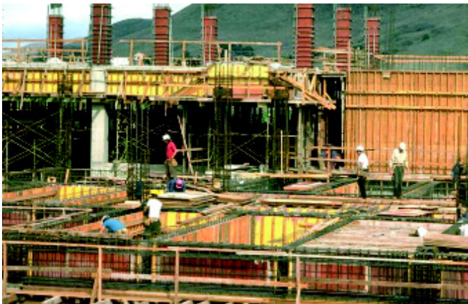
Improving our infrastructure is one solution towards addressing today's social, economic and environmental problems.
